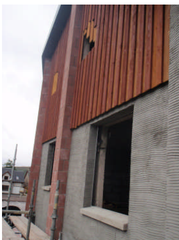
Fig. 6 : Openings in eastern elevation
